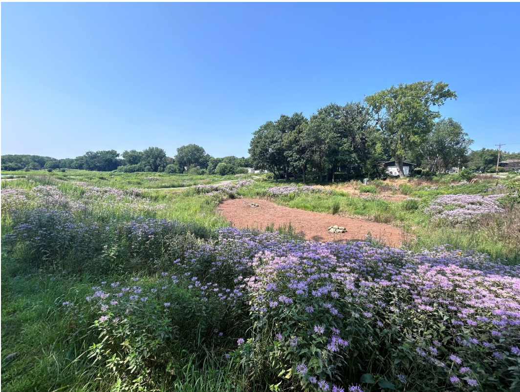
Figure 4 Hansen Park, Iron Enhanced Sand Filter, New Brighton, MN
