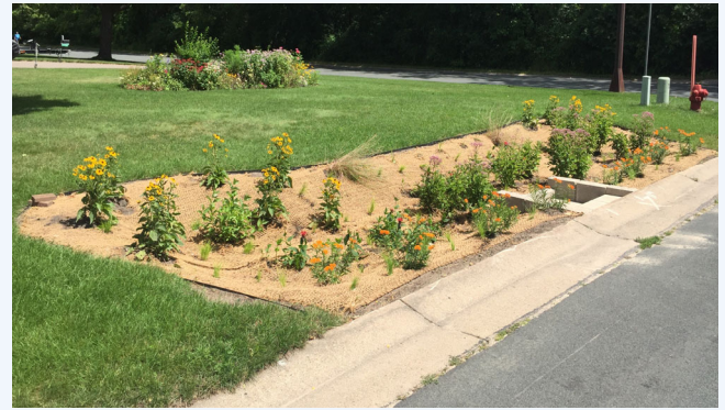
Recently installed raingarden
