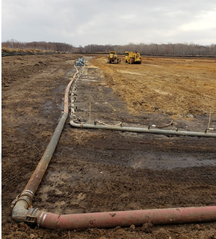
Figure 12 Construction Dewatering Site
