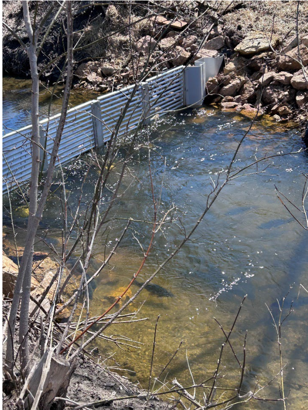
Figure 6 Johanna Creek Carp Barrier, New Brighton MN
