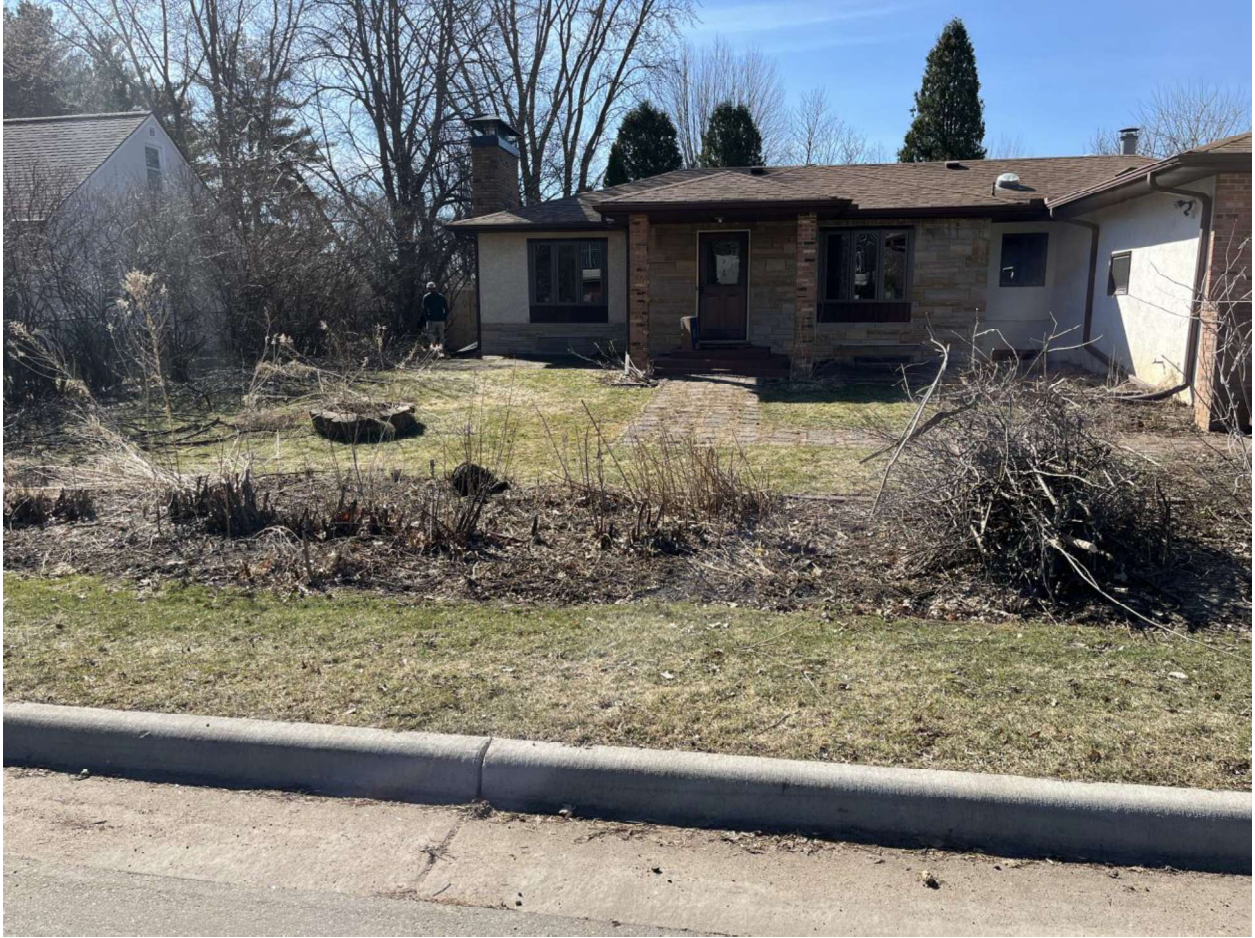
PRE-EXISTING CONDITIONS PHOTO 1 OF 2
