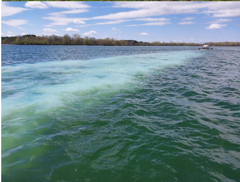
Centerville Lake Alum Project. Top: Staging site set-up, with temporary shoreline storage tanks Bottom: Alum application, April 28, 2026
