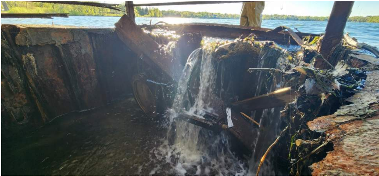
Photo 7: Knife Gate & Broken Sheet Pile Cap
