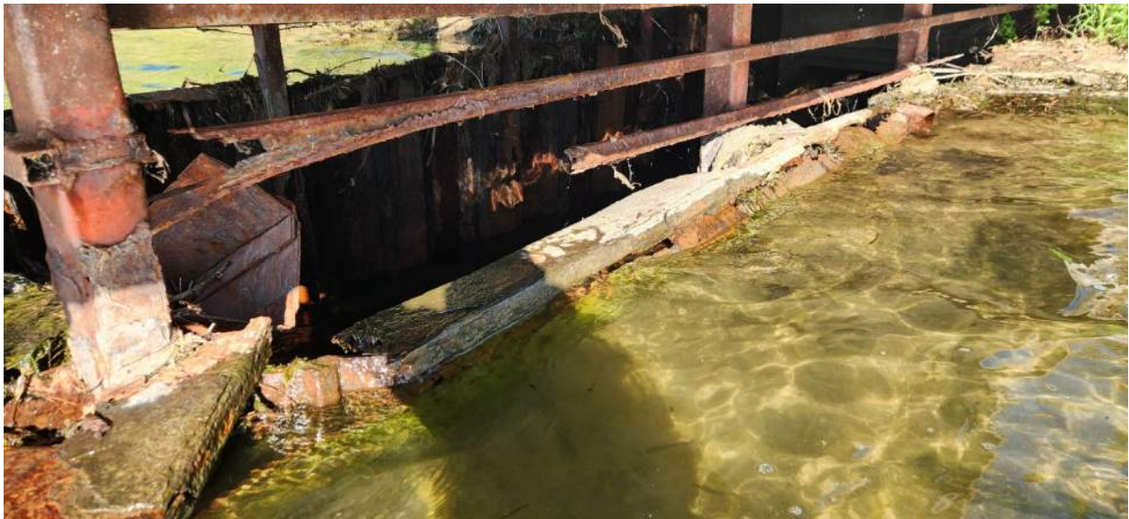
Photo 6: Broken Underside Railing
