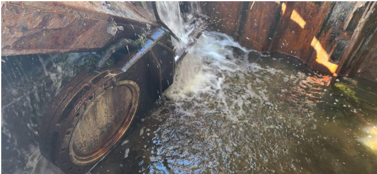
Photo 8: Knife Gate & Broken Sheet Pile Cap
