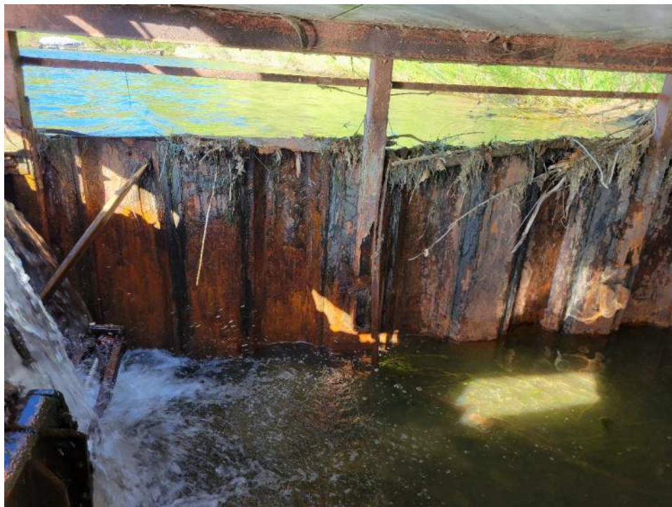
Photo 2: Rotted Post Supports
