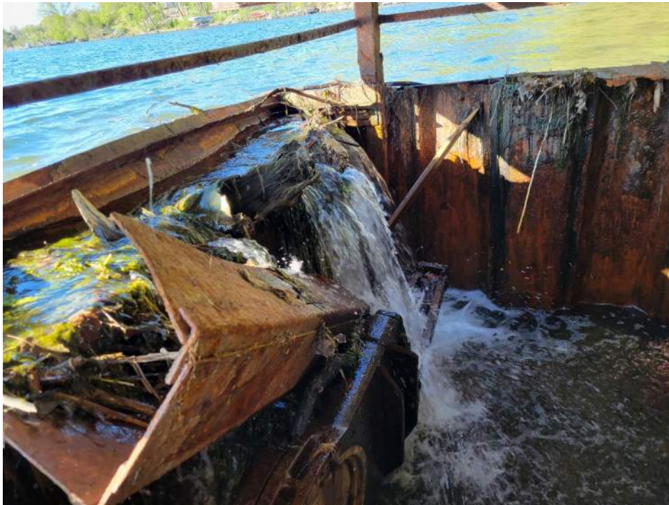
Photo 9: Debris Skimmer & Sheet Pile Cap
