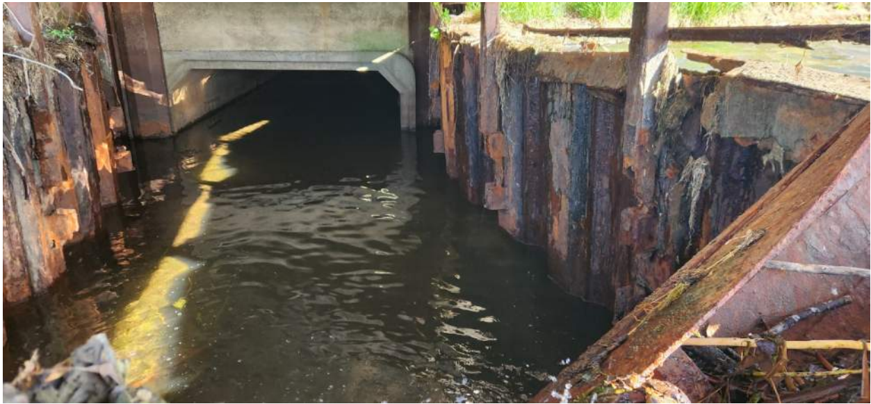
Photo 5: Rotted Post Supports
