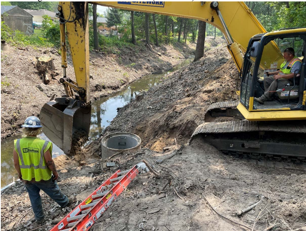
29. Backfilling manhole with ONSITE sand (12:35 PM).
