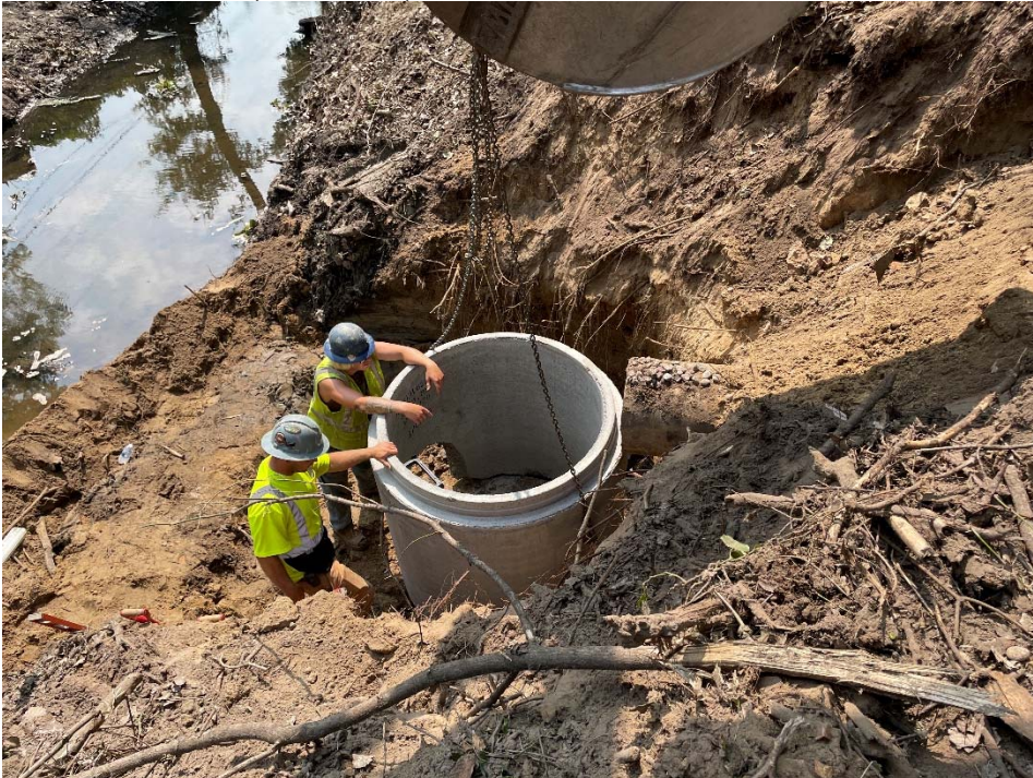
25. Placing Manhole (11:30 AM)
