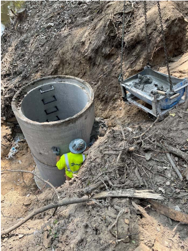
27. Nate sealing upstream pipe with concrete (12:15 PM)
