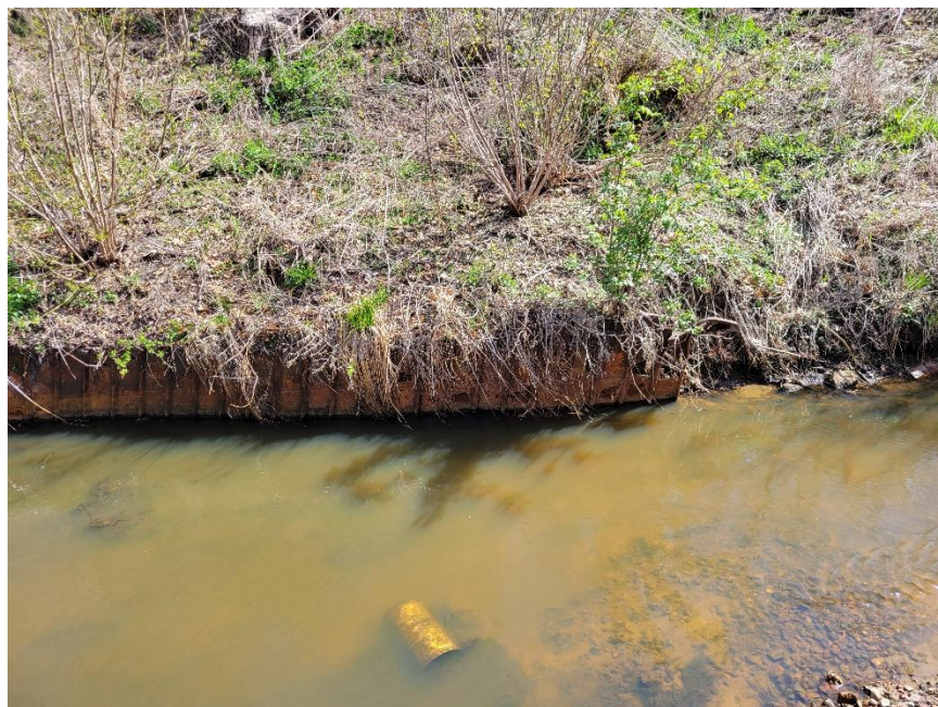
Photo 6- Bank Conditions Across from Pipe Outlet
