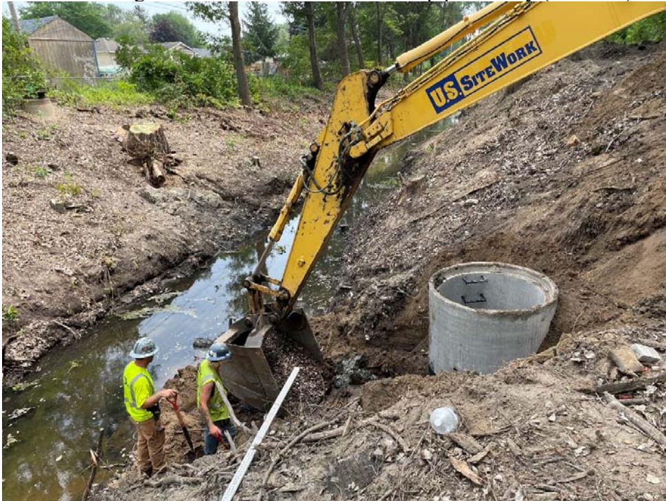
31. Nicholas adding rock below where downstream pipe will lay (1:20 PM).
