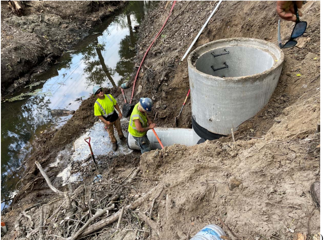
37. Pipe with gasket on it (4:00 PM).
