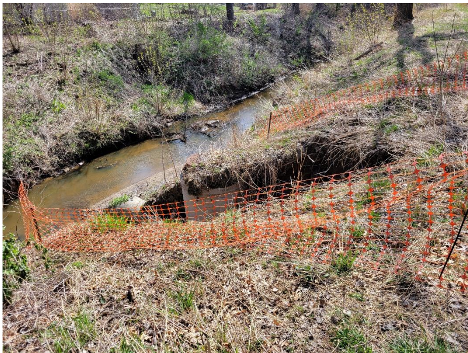
Photo 1: Scour/erosion area
