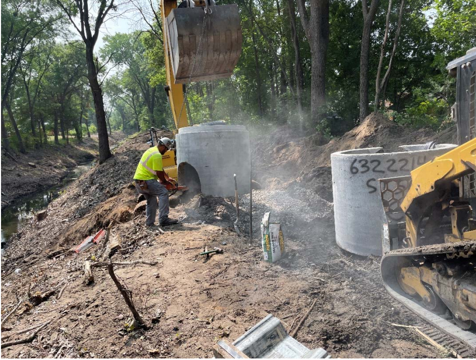
25. Placing Manhole (11:30 AM)
