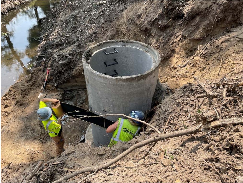
29. Backfilling manhole with ONSITE sand (12:35 PM).
