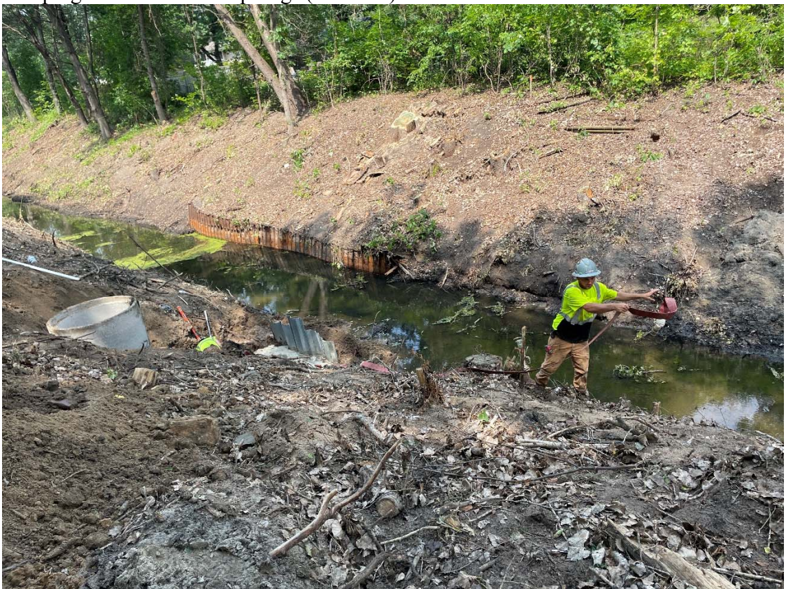
33. Pumping out water behind pilings (2:00 PM).
