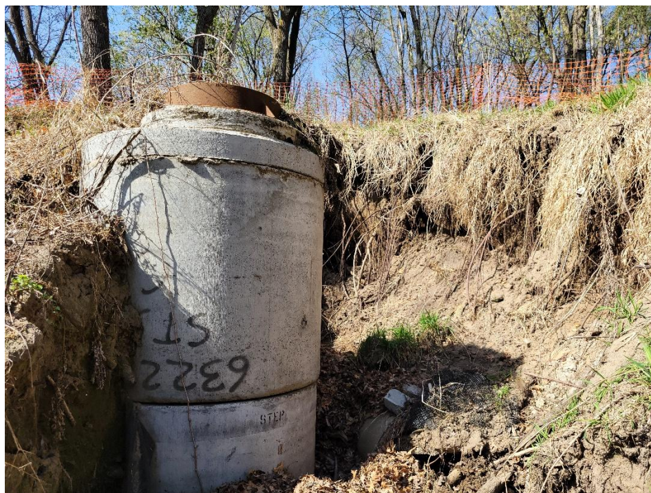
Photo 2: Scour/erosion area
