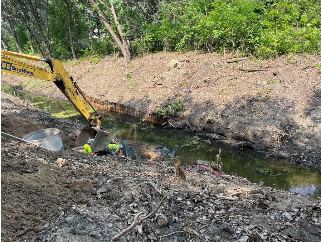
35. Finished cutting pilings (3:30 PM).
