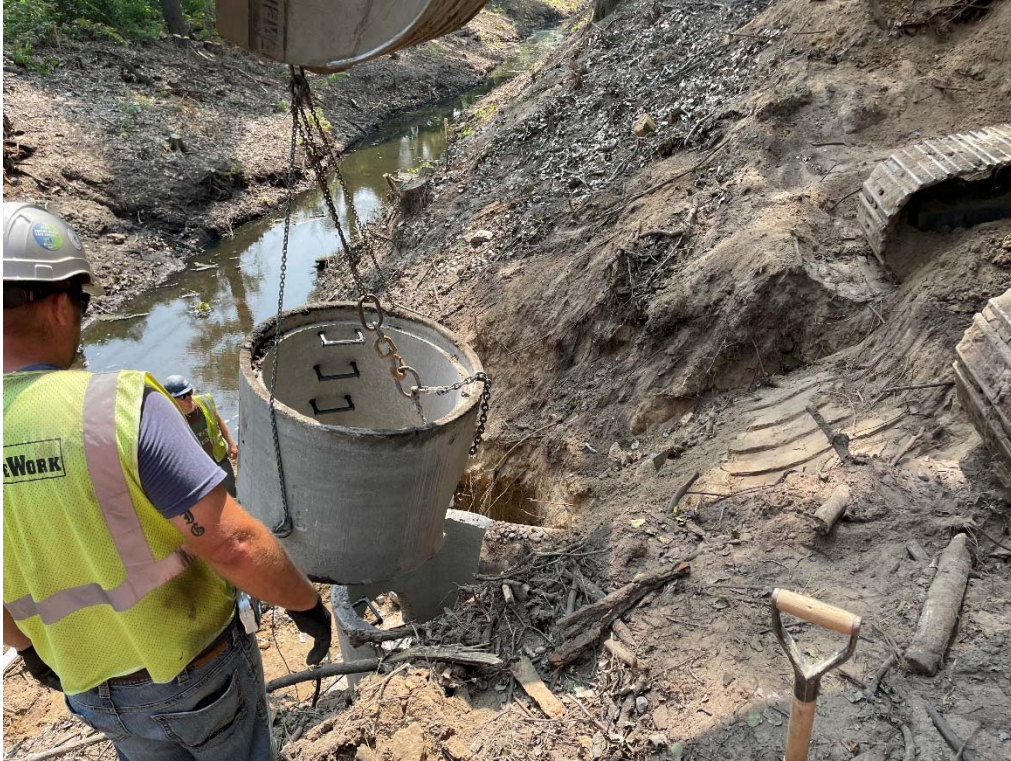
27. Nate sealing upstream pipe with concrete (12:15 PM)
