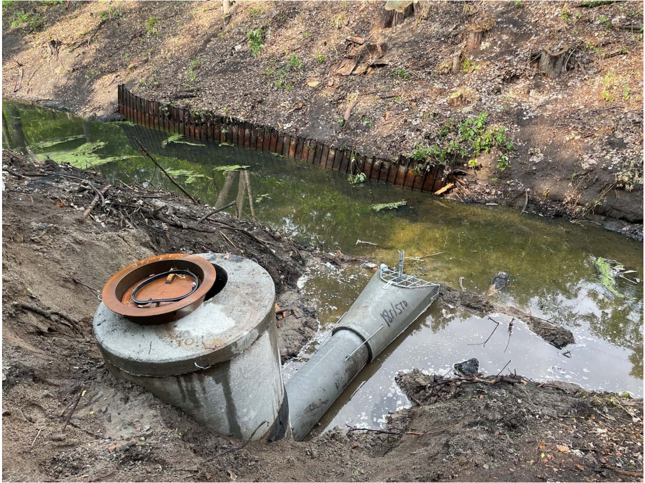
38. Site at the end of the day (5:00 PM).
