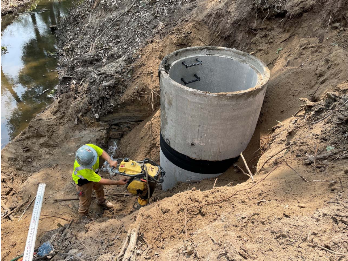
31. Nicholas adding rock below where downstream pipe will lay (1:20 PM).
