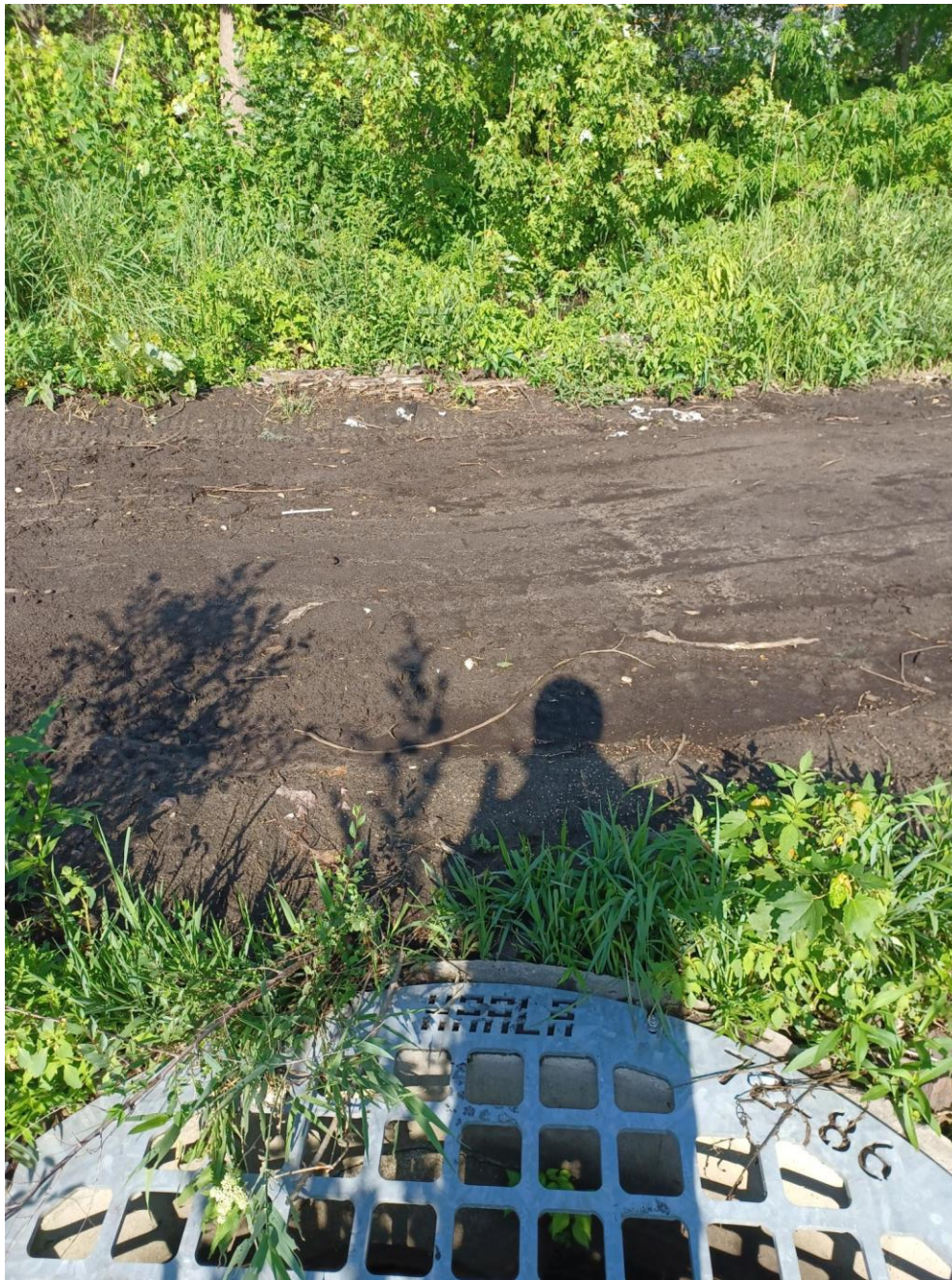
Photo #3: Manhole and storm apron to protect near STA 26+00
