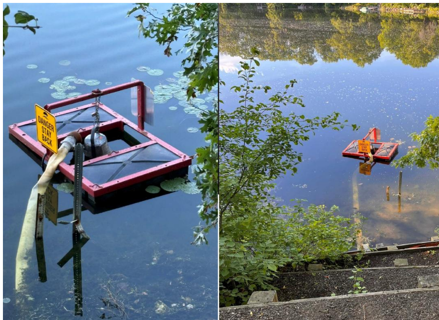
Figure 1. The current Karth Lake overflow pump, manually deployed and operated
