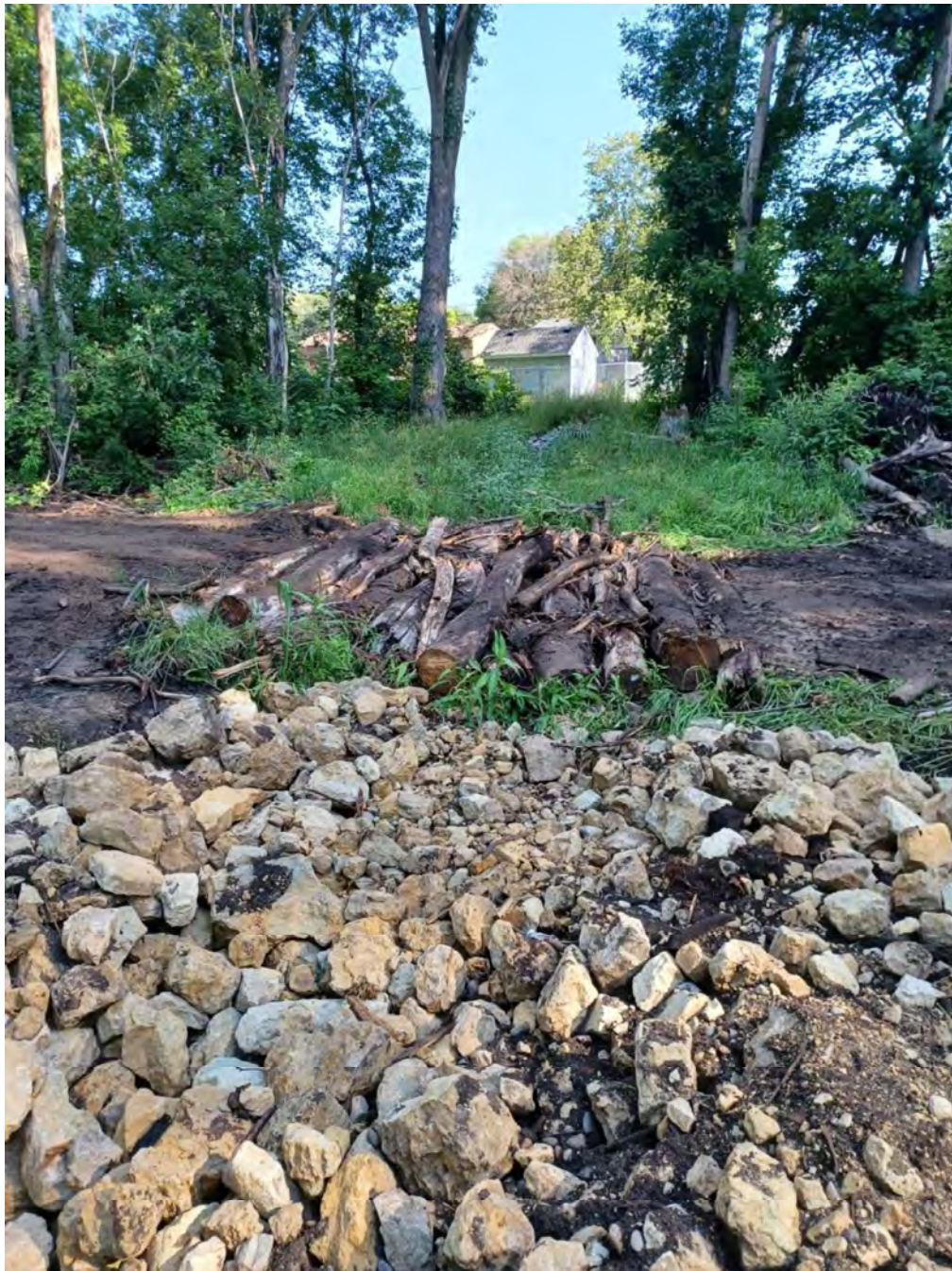
Photo #5: More logs to be removed near STA 33+00
