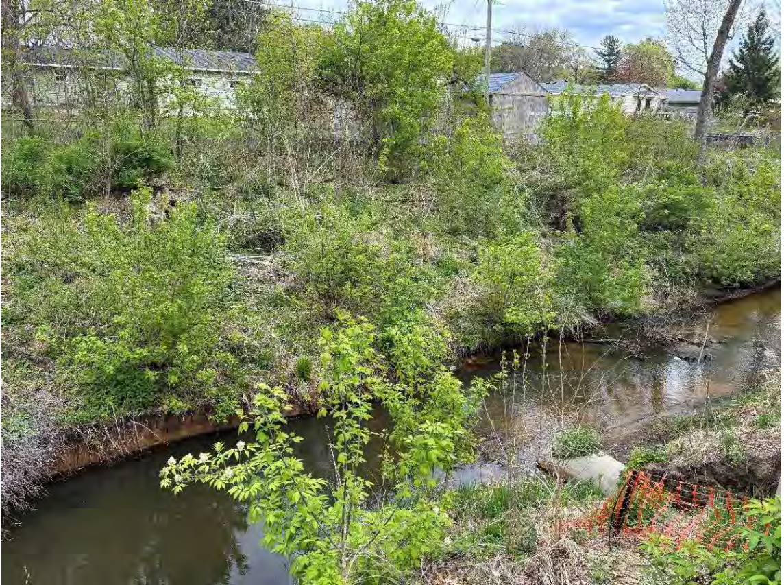
Figure 2. Debris Accumulation and Vegetation Growth in Trash Guard
