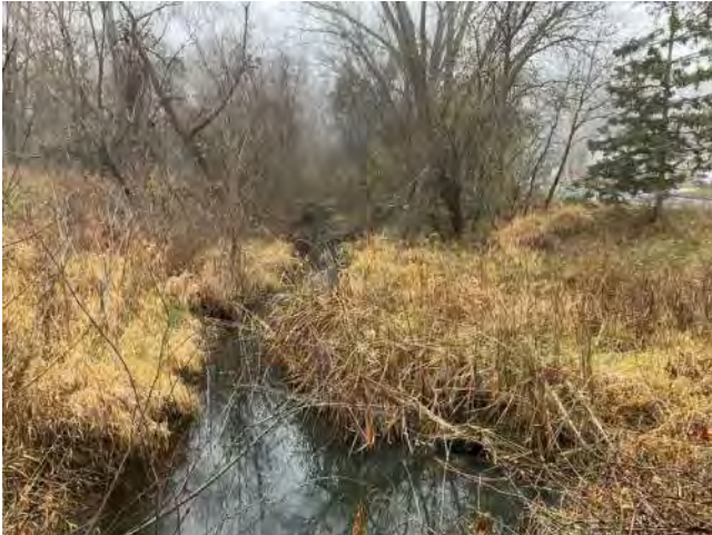
Photo #2: Heavy Vegetation in ditch, Main Trunk STA: 53+00
