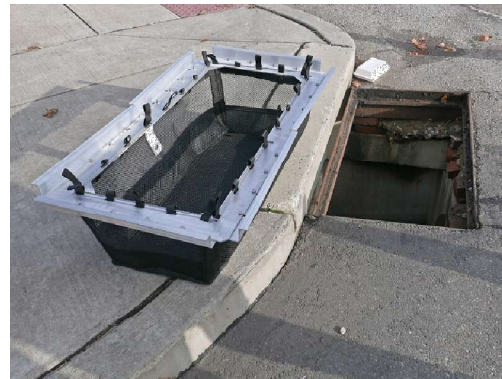
StormSack is a geotextile catch basin insert
