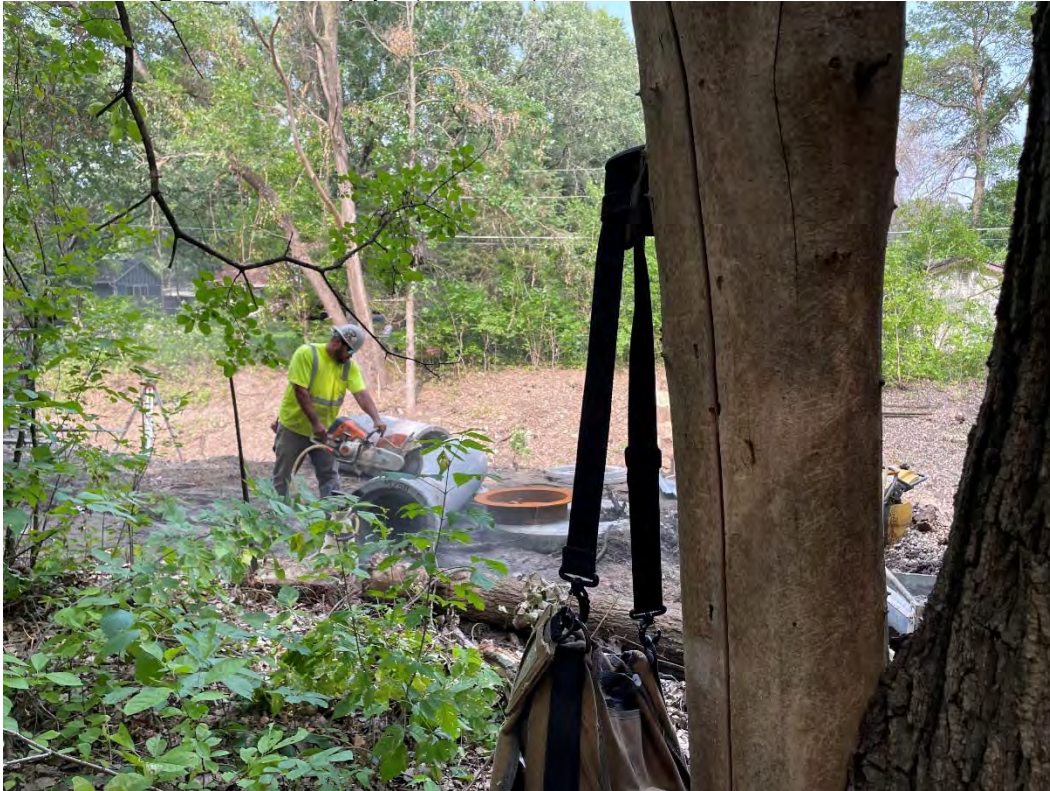
36. Justin cutting downstream pipe (3:40 PM).
