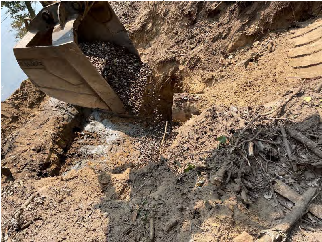
19. Nicholas adding rock to manhole base area (10:50 AM).
