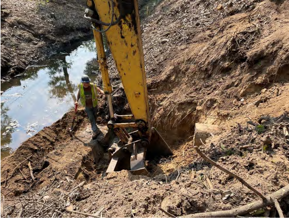
19. Nicholas adding rock to manhole base area (10:50 AM).
