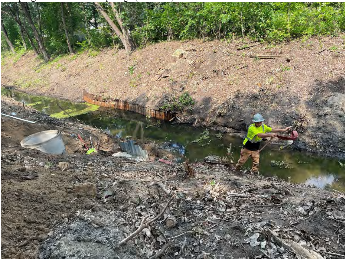
33. Pumping out water behind pilings (2:00 PM).
