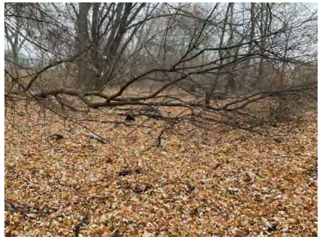
Photo #12: Deadfall in channel, Branch 5 STA: 17+00
