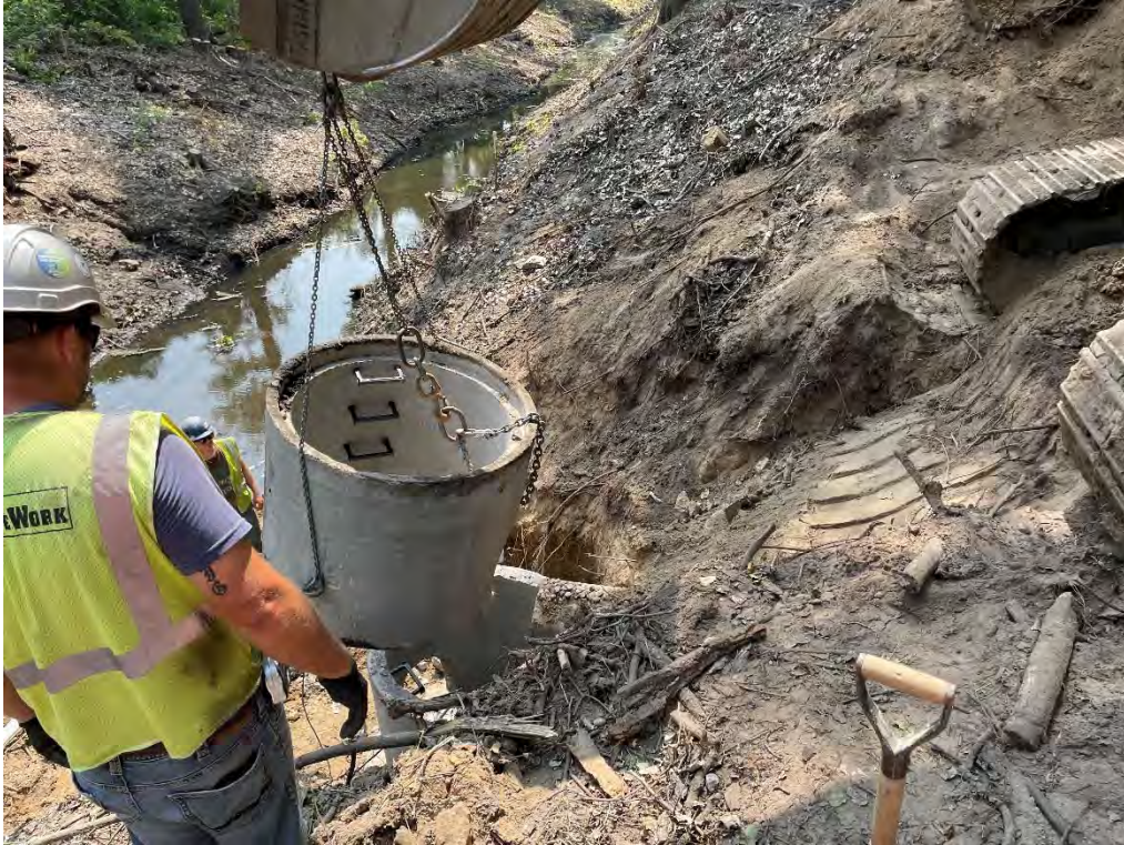
27. Nate sealing upstream pipe with concrete (12:15 PM)
