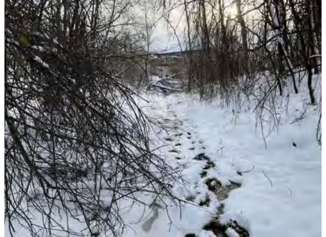
Photo #11: Deadfall in channel, Branch 3 STA: 1+00
