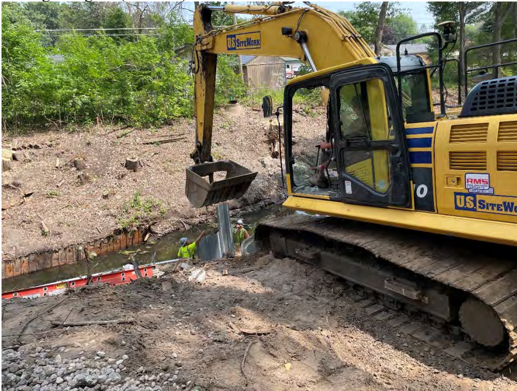
33. Pumping out water behind pilings (2:00 PM).
