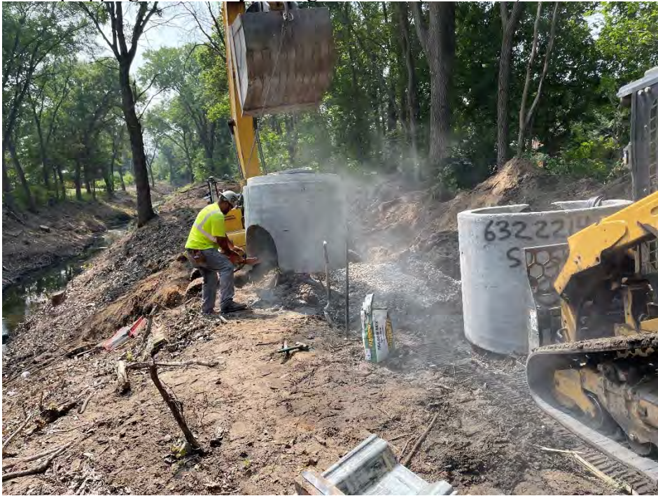
25. Placing Manhole (11:30 AM)
