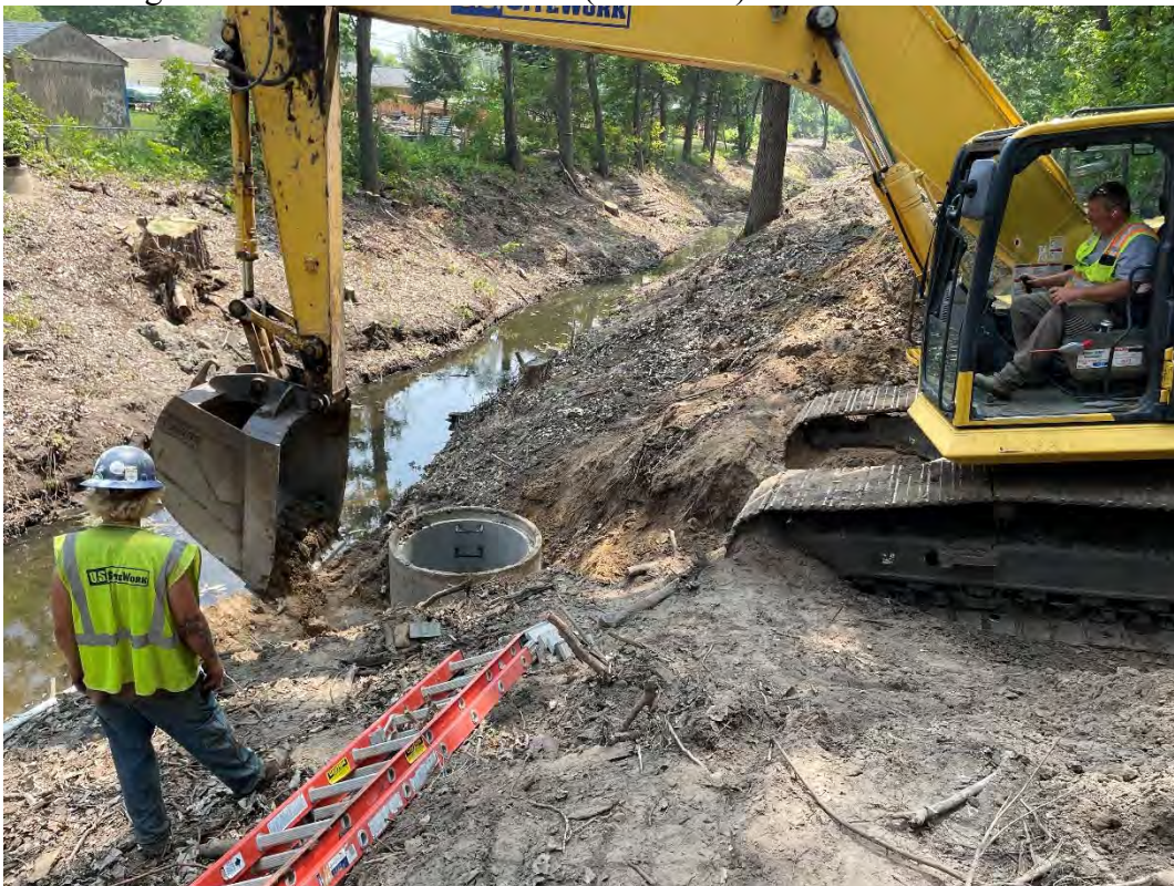
29. Backfilling manhole with ONSITE sand (12:35 PM).
