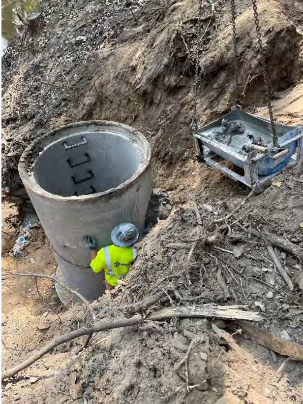
27. Nate sealing upstream pipe with concrete (12:15 PM)
