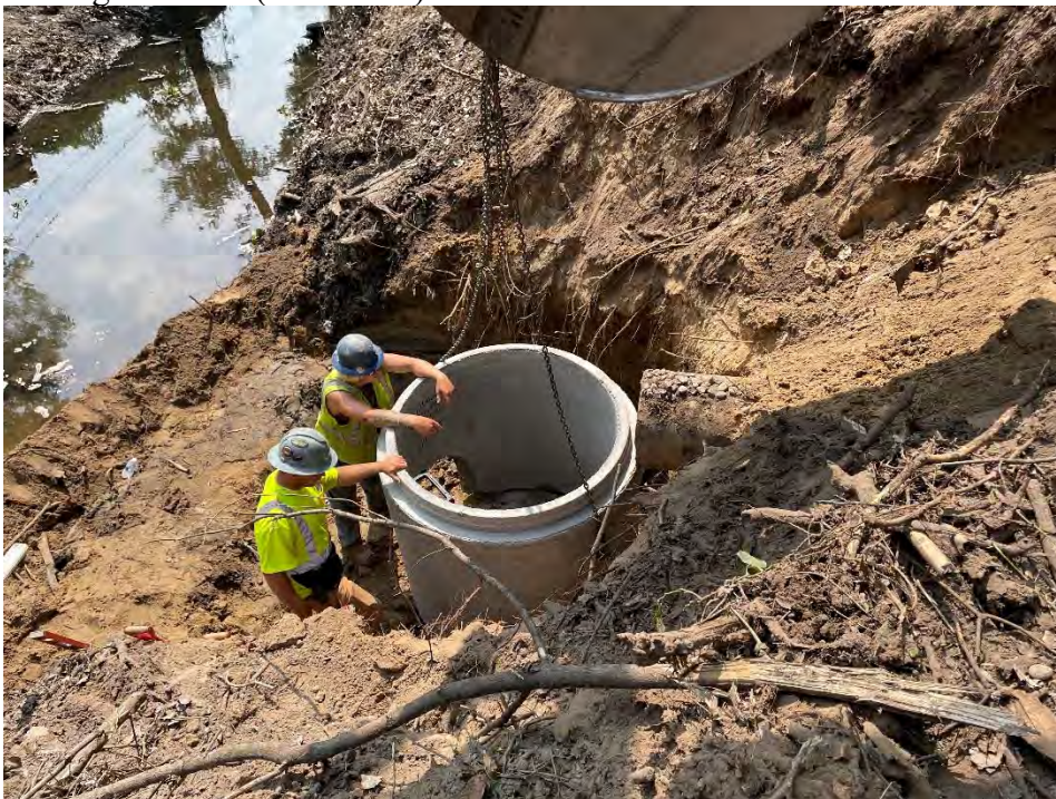
25. Placing Manhole (11:30 AM)
