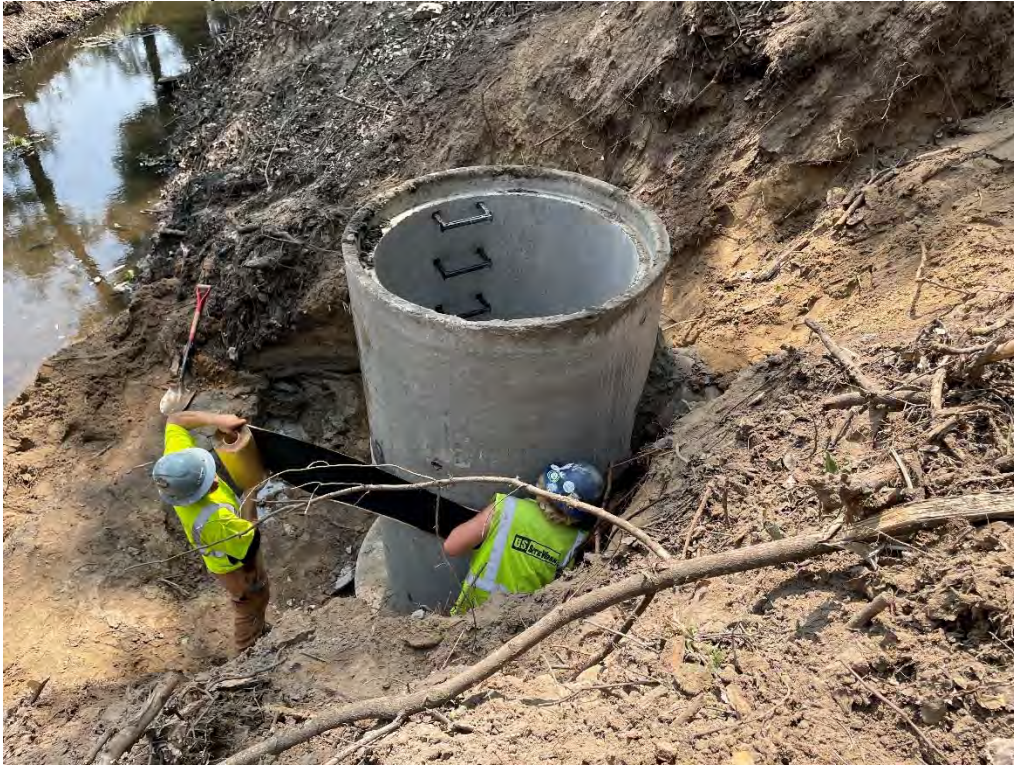
29. Backfilling manhole with ONSITE sand (12:35 PM).
