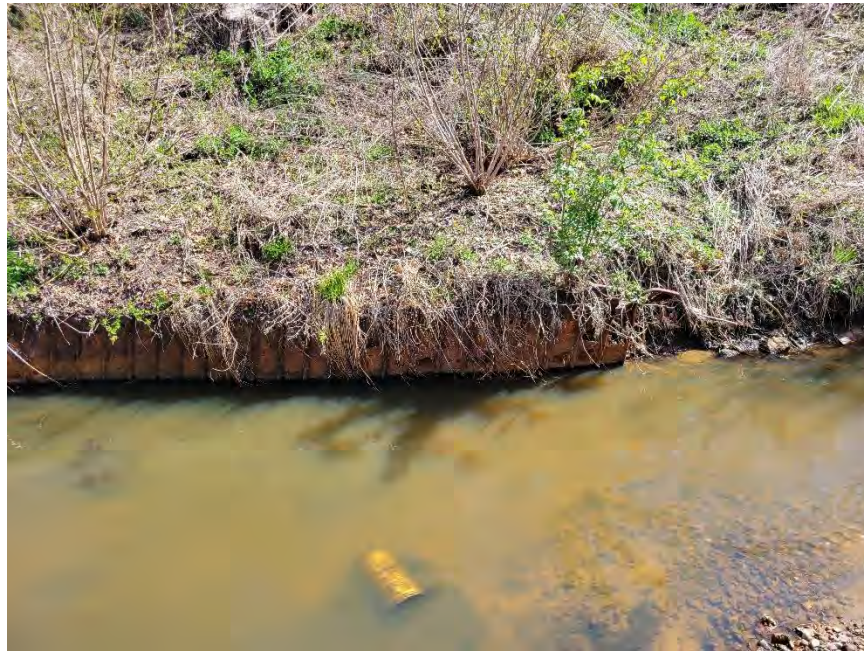
Photo 6- Bank Conditions Across from Pipe Outlet
