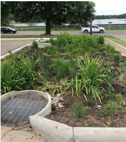
Completed raingarden in Shoreview
