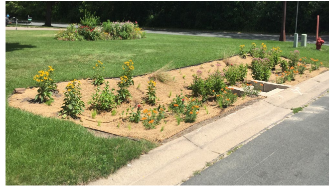
Recently installed raingarden
