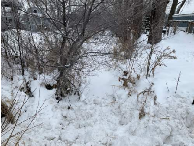
Photo #9: Ditch next to mobile homes, Branch 2 STA: 61+50
