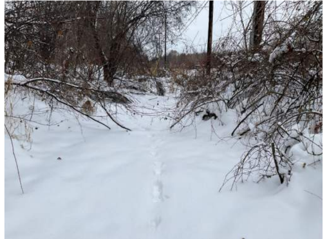
Photo #7: Overhead Power Lines next to ditch, Branch 2 STA: 33+50
