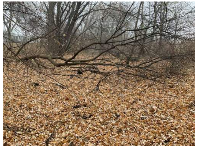
Photo #12: Deadfall in channel, Branch 5 STA: 17+00
