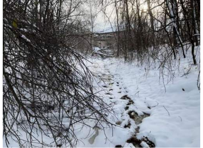
Photo #11: Deadfall in channel, Branch 3 STA: 1+00
