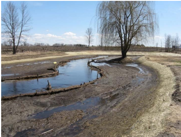
Figure 2. Streambank stabilization site immediately following construction
