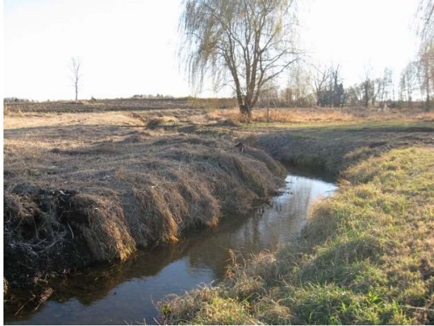
Figure 1. Streambank stabilization site, prior to restoration
